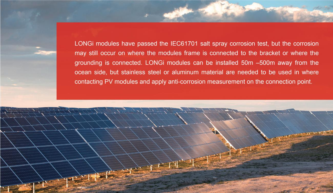
LONGi modules have passed the IEC61701 salt spray corrosion test, but the corrosion may still occur on where the modules frame is connected to the bracket or where the grounding is connected. LONGi modules can be installed 50m –500m away from the ocean side, but stainless steel or aluminum material are needed to be used in where contacting PV modules and apply anti-corrosion measurement on the connection point.
